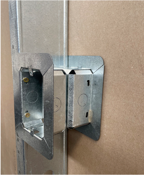
Acoustic Flush Box Installation
